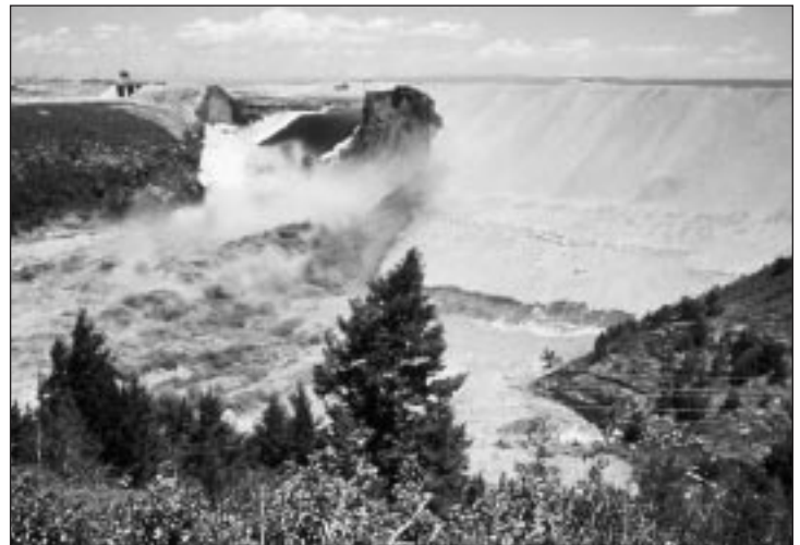
On June 6, 1976 the Teton Dam near Rexburg, Idaho failed during its initial filling. The deluge killed at least 11 people. At 350 feet high, it was the largest dam break in US history. Damages reached $1 billion.
