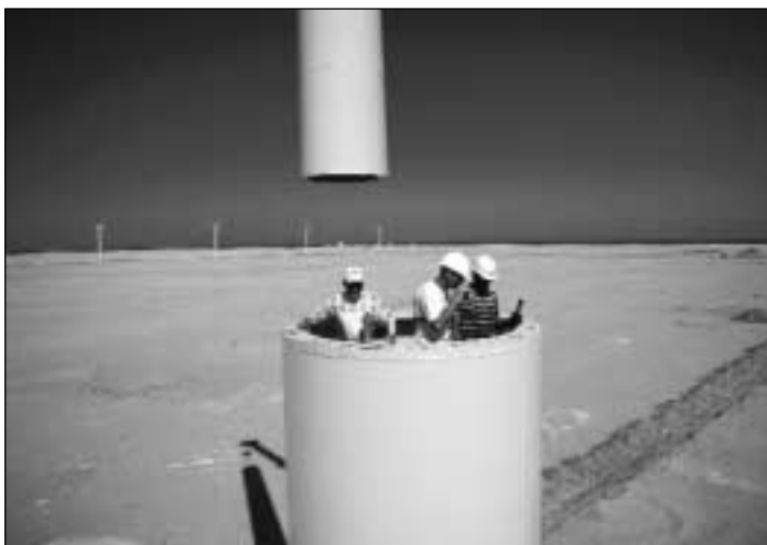
Installing wind turbines in Egypt.
