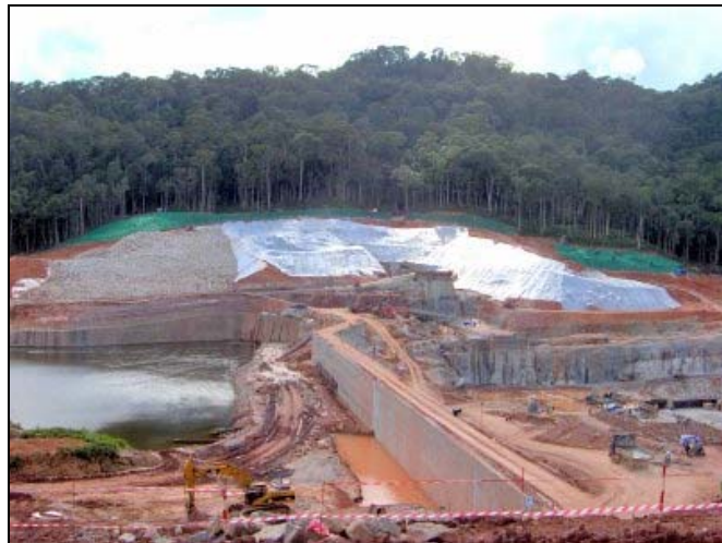
Photo 1: Nam Theun 2 dam construction site.
