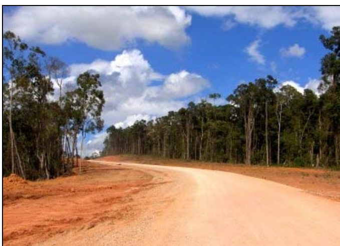
Photo 10: Road construction in the NT2 Corridor.
