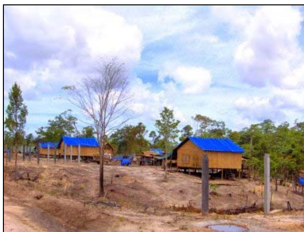
Photo 5: New temporary housing at Ban Boua Ma resettlement village.
