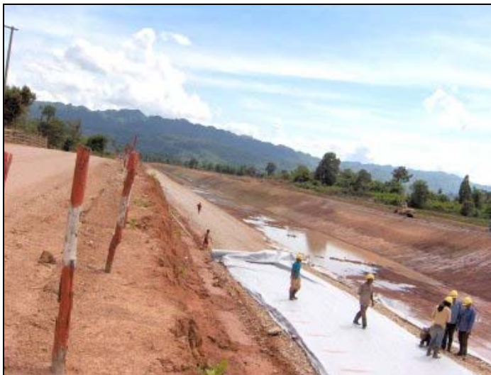
Photo 2: The downstream channel, which will carry water from the powerhouse to the Xe Bang Fai.
